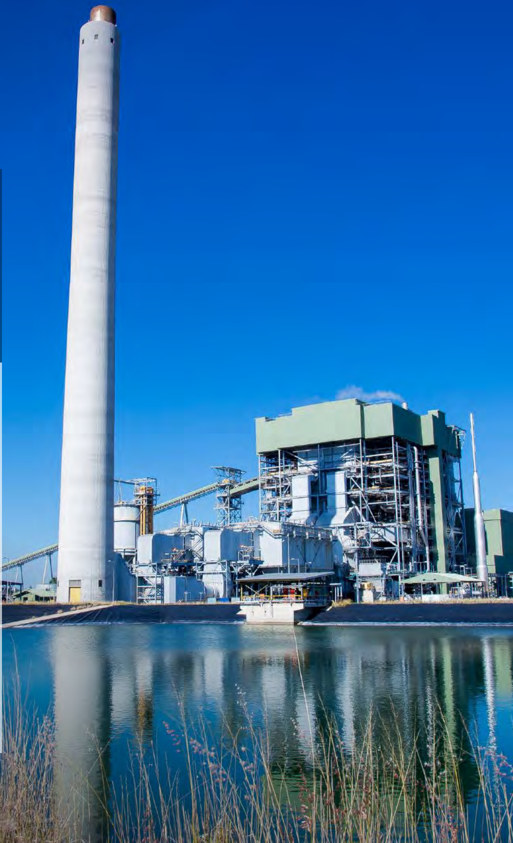
Photo: Kogan Creek Power Station operated at 95 per cent availability in FY2019.
